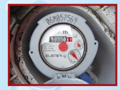
This meter has 3 red numbers at the end- they show hundreds, tens and units of litres. The dial shows centilitres, so the meter reading here is a 70,812 litres and a few millilitres.
